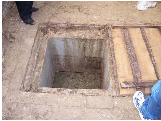
Figure 6. Biogas pits in a) Shangri-la (Yunnan Province) and b) Inner Mongolia, June 2005. The end product of biogas production, called biogas slurry, makes excellent organic fertilizer.
