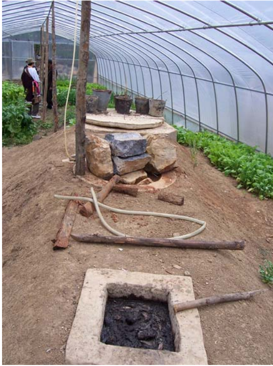
Figure 6. Biogas pits in a) Shangri-la (Yunnan Province) and b) Inner Mongolia, June 2005. The end product of biogas production, called biogas slurry, makes excellent organic fertilizer.
